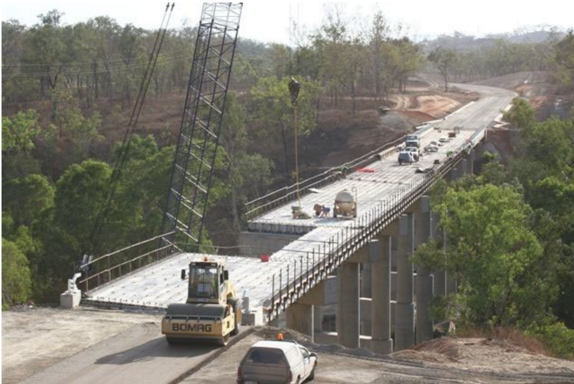
Building of the West Normanby River Bridge
